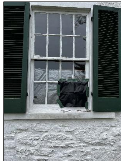
Boarding Up Broken Windows
