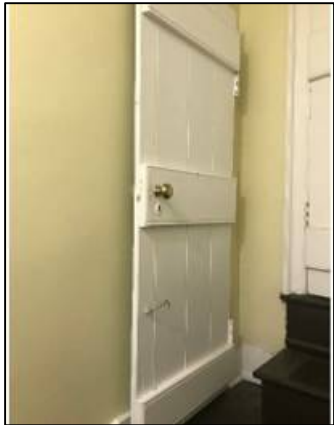
Relocation of Original Door
