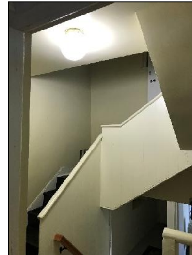
Replacing Bulbs & Fixtures
